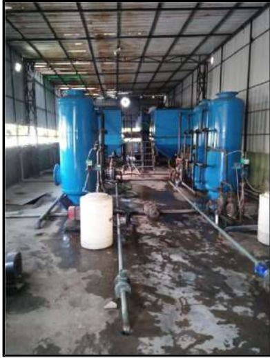
Sewage Treatment Plant
